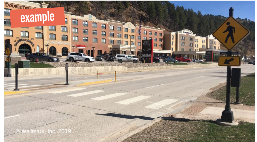
Example of an enhanced pedestrian crossing with RRFBs from Deadwood, South Dakota.
