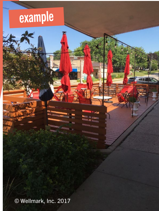
This parklet was installed next to a restaurant to provide outdoor dining space for customers.
